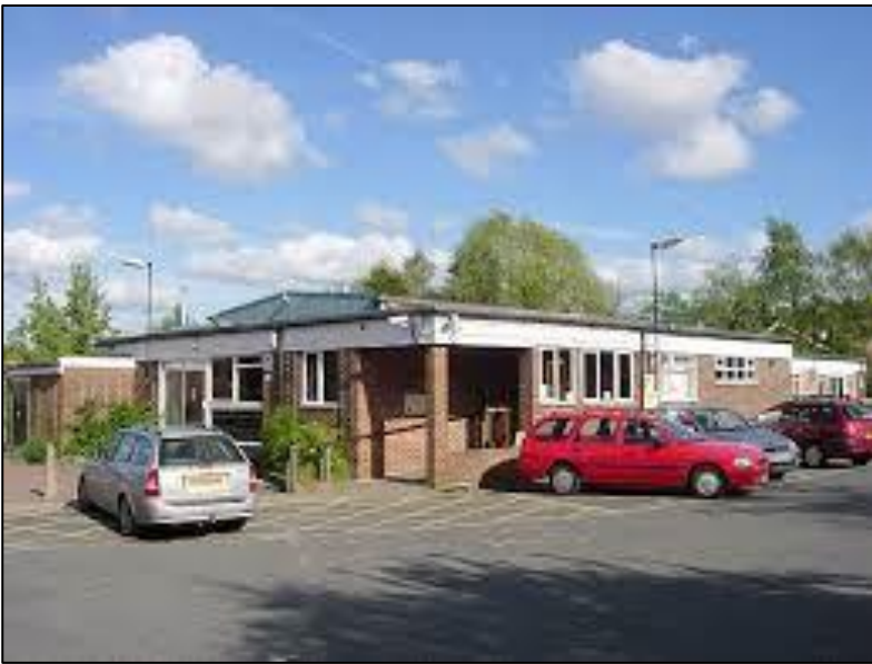
Sevenoaks Community Centre entrance circa 1999
