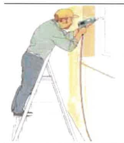
Correct – steps facing work activity
