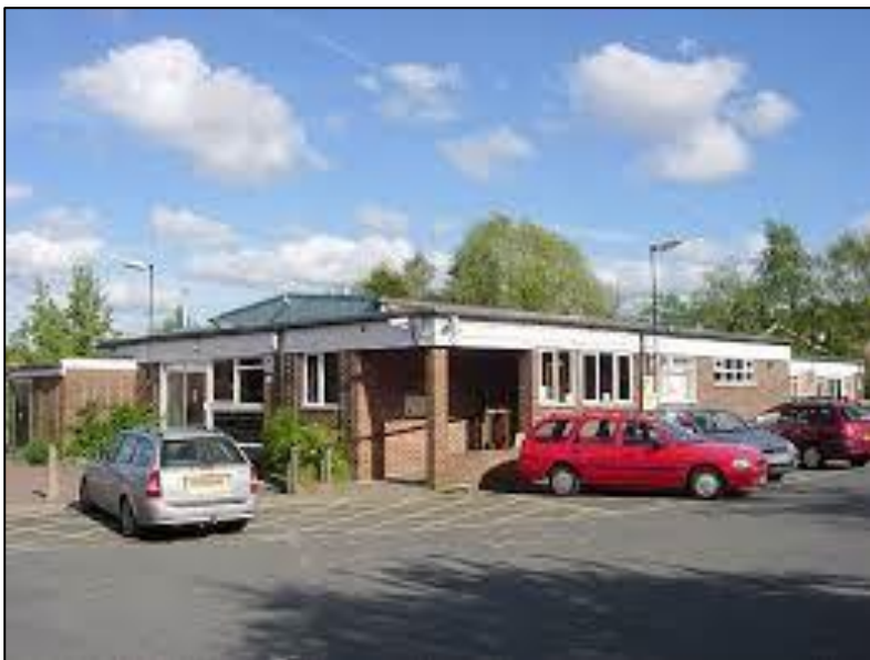
Sevenoaks Community Centre entrance circa 1999
