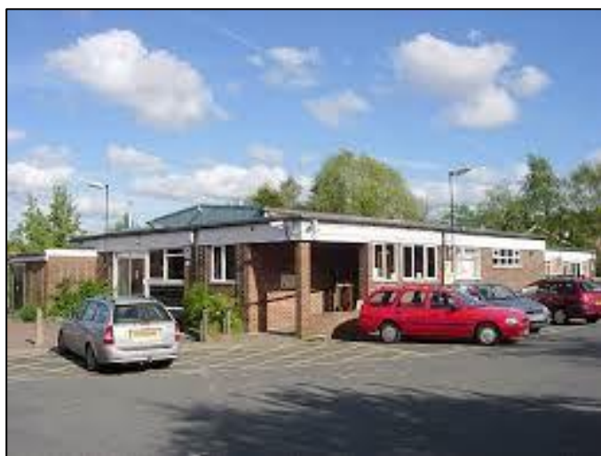
Sevenoaks Community Centre entrance circa 1999
