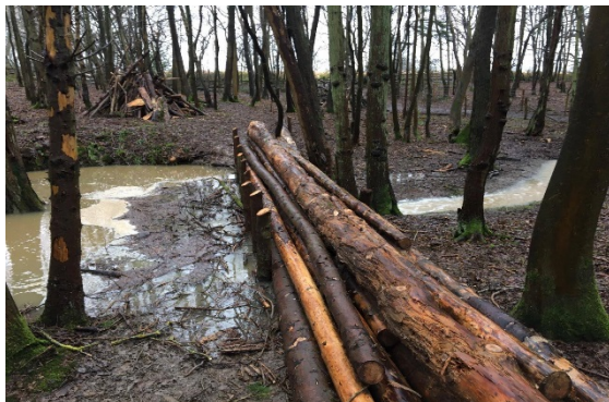
Above and right: leaky woody dams installed by the NFM pilot project
