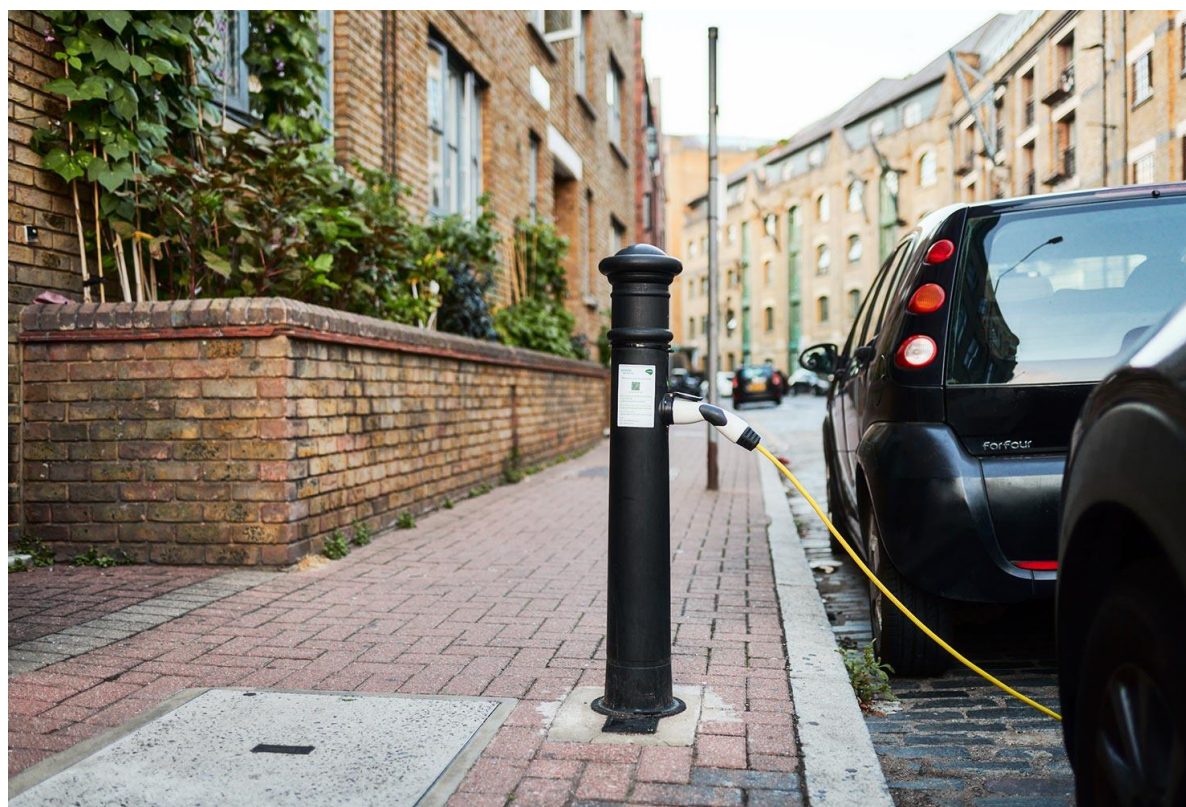
Figure 2, Example of Bollard Charge point
