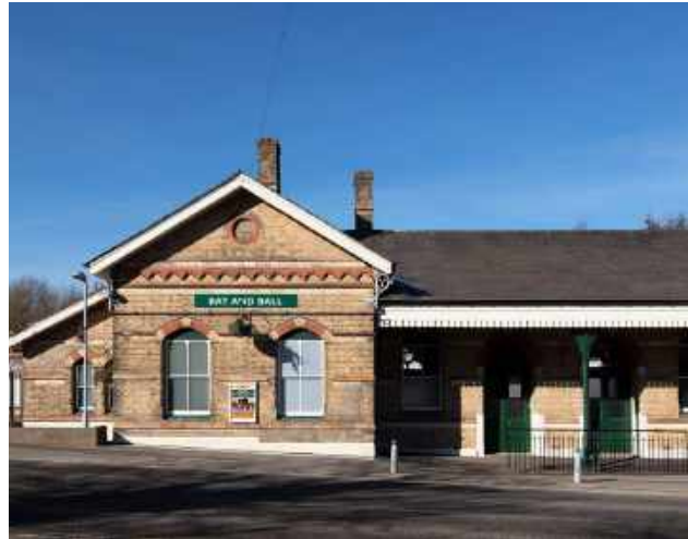
The recently refurbished Bat and Ball station building
