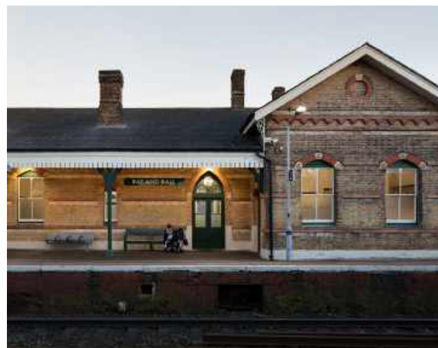
The recently refurbished Bat and Ball station provides a more welcoming arrival experience into the town
