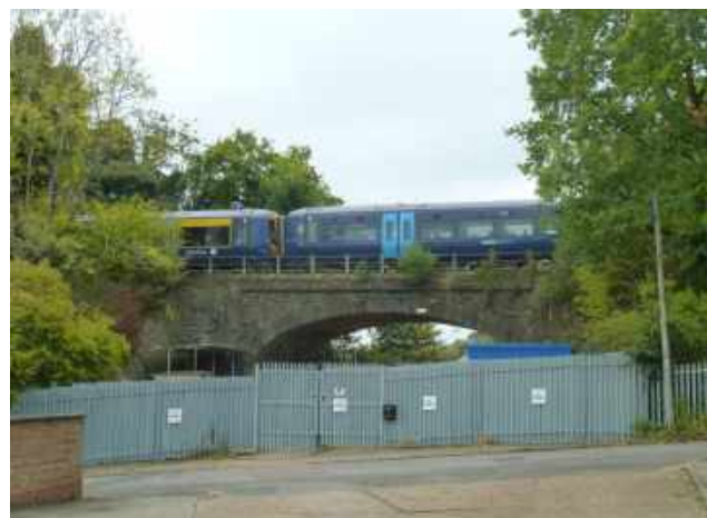
FROM TOP: Poor street environment at Sevenoaks station; access under the rail line blocked for pedestrians to the north of the station
