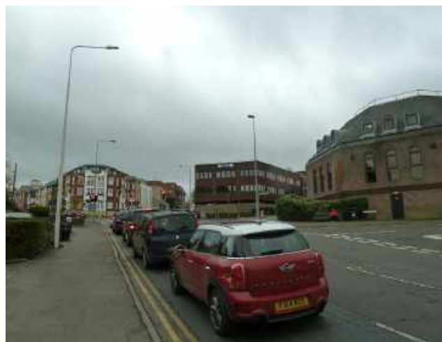
Offices on London Road / Argyle Road
